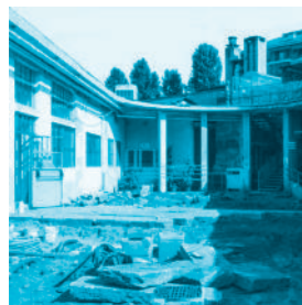
> Co-City building site Photo Beeozanam
